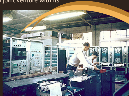
LEO III/2 being commissioned at Minerva Rd. before being shipped to Johannesburg. L. to R. Lou Weatherill and Frank Wroe. Senior Commissioning Engineer, Tony Morgan.
